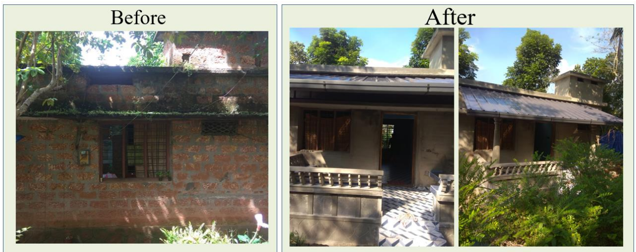
Figure 2: House repair at Ms. Lissy PP
